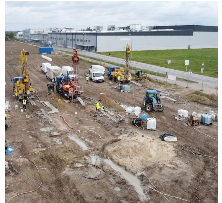
Sieradz expansion ground heating wells.
