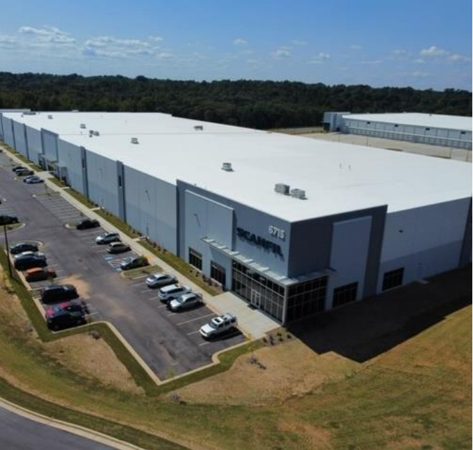
Atlanta factory expansion in The USA
